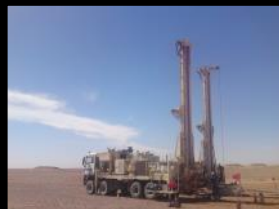
Mobile Drill Rig
